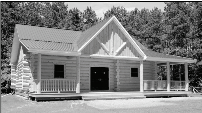
The new Limerick Forest Interpretive Centre. Photo by Valerie Kirkwood.
