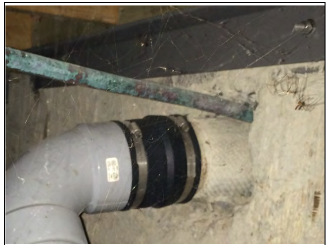
Photo 4: Presumed asbestos-containing cement pipe observed to be in good condition in the crawlspace.
