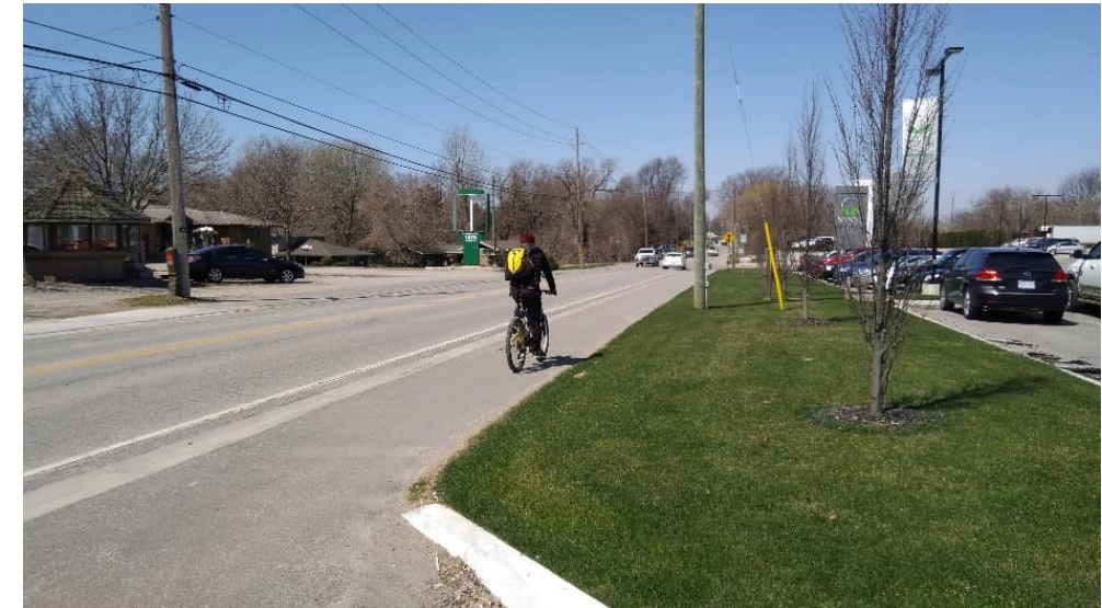
Figure D-8: A maintenance strip repurposed as a shared walking and cycling facility in Essex County, ON
