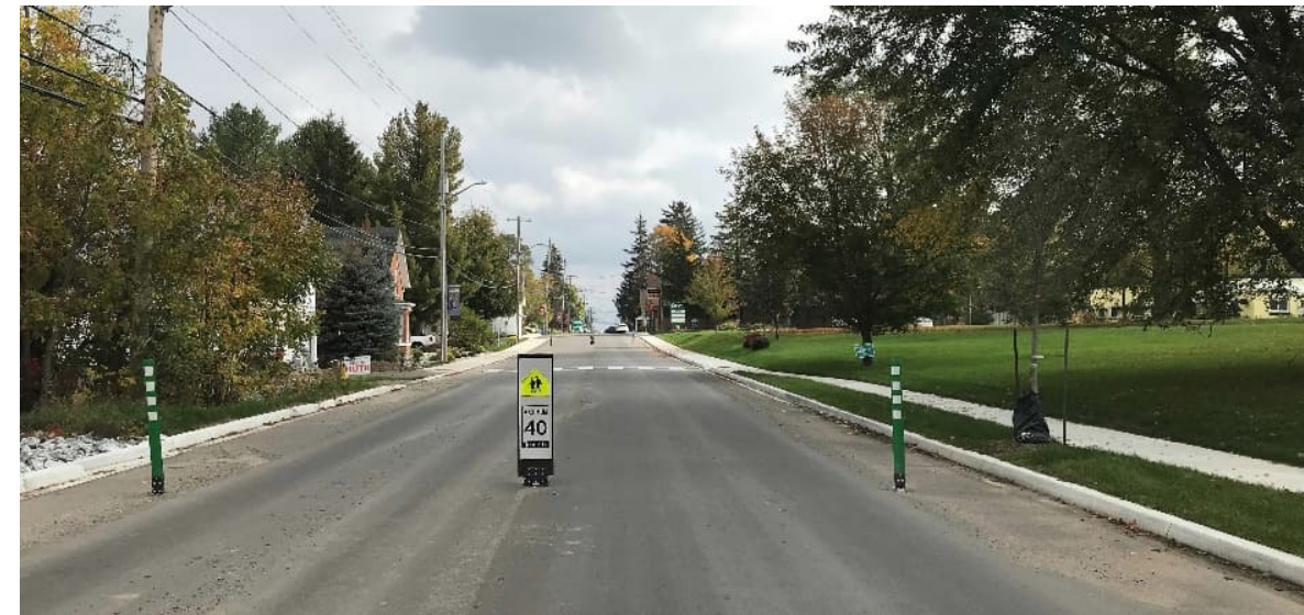
Figure D-16: Traffic calming measures in advance of pedestrian crosswalk on Bedford Street, Westport
