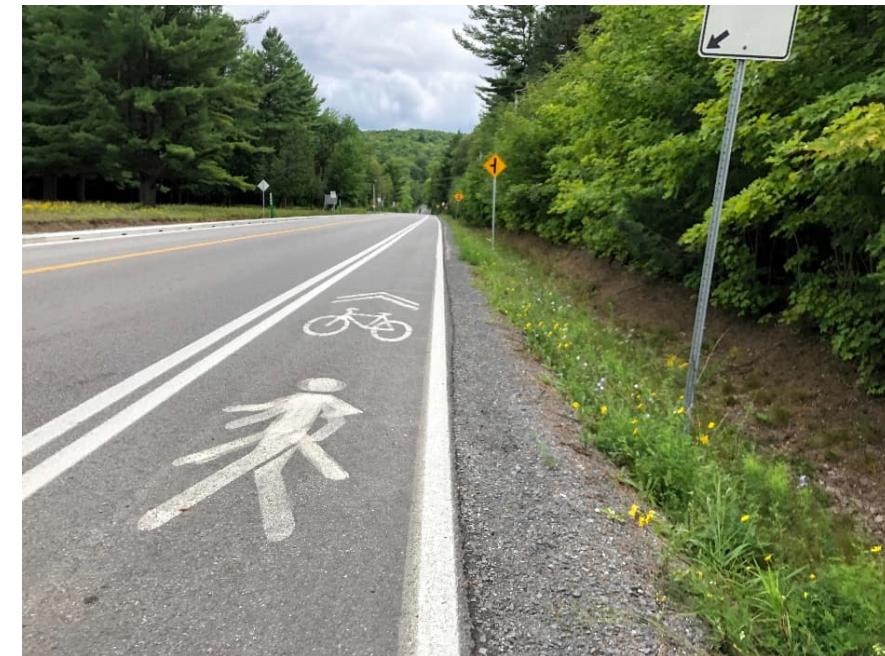
Figure D-6: A paved shoulder designated for pedestrians and cyclists in Gatineau, Quebec
