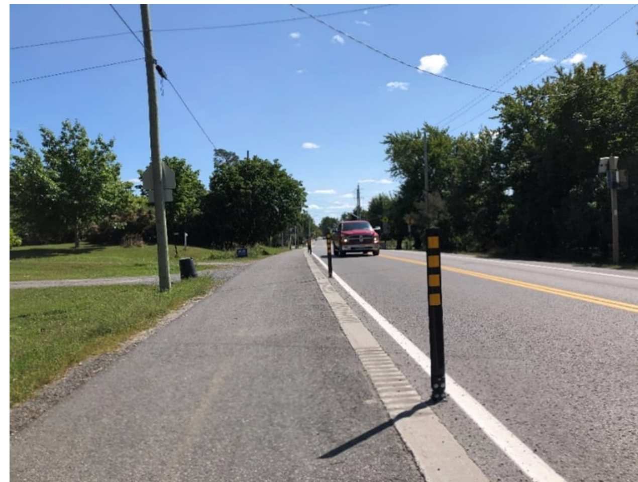
Figure D-9: Delineator posts separating a multi-use pathway from traffic in the village of Kars in Ottawa
