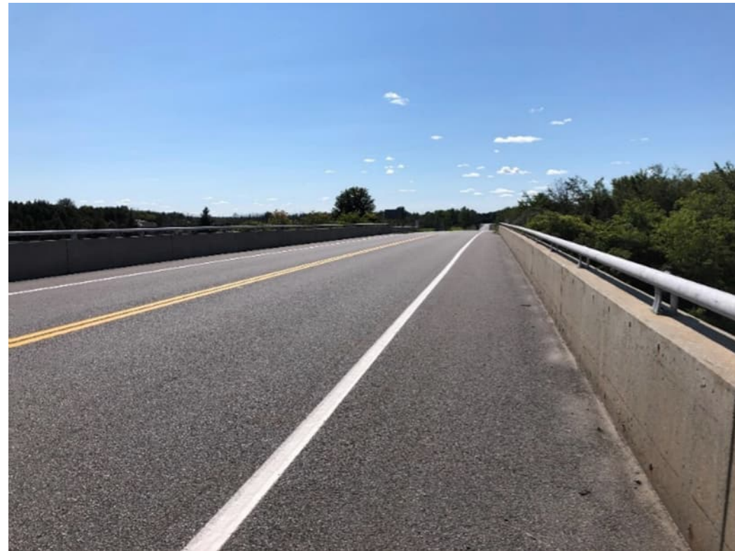
Figure D-4: Paved shoulder extended over a bridge in Ottawa, ON
