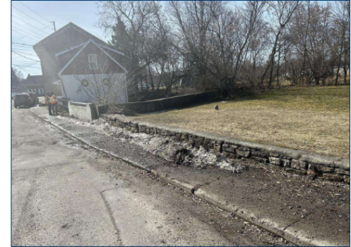
Photo 3 – Retaining wall(s) – West Side
