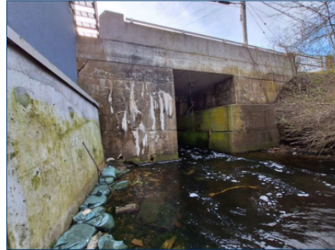
Photo 2 – East Side of Structure
