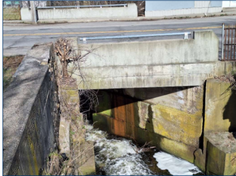
Photo 1 – West Side of Structure
