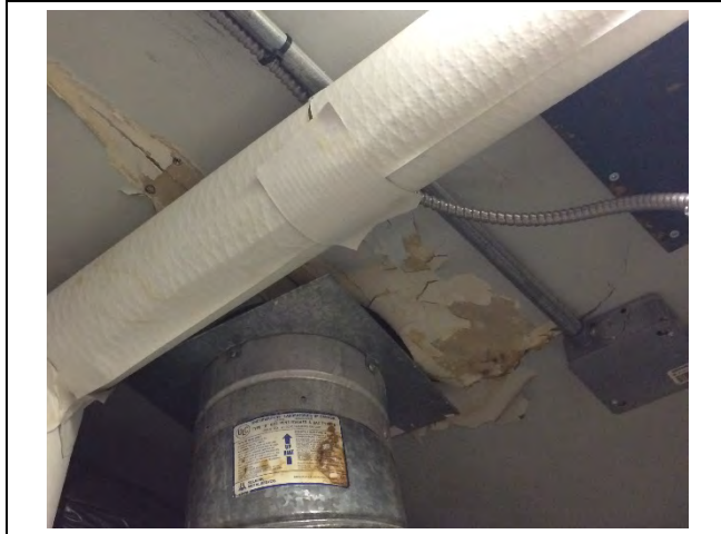
Photo 1: Asbestos-containing drywall joint-fill compound observed to be in poor condition on the ceiling in the hot water tank room located in the laundry room.
