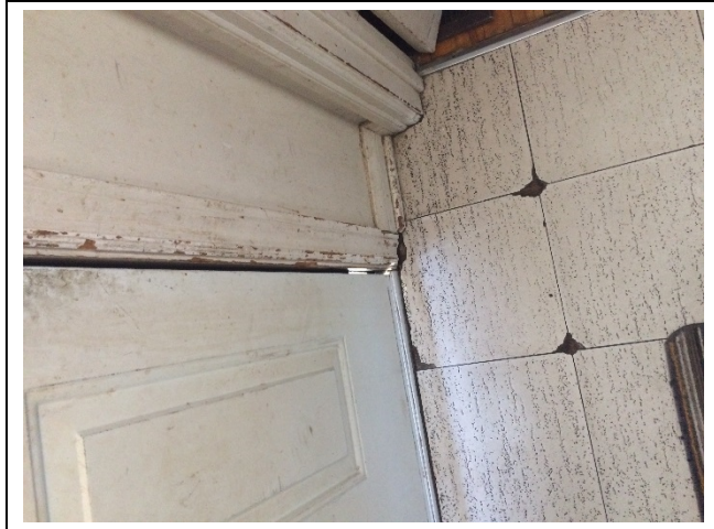
Photo 1: Asbestos-containing 12"x12" vinyl floor tiles – beige with black dots in the foyer of 116 Brighton Crescent.
