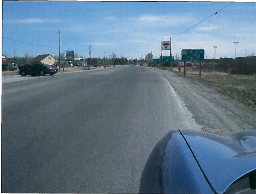
West of Wellington Street
