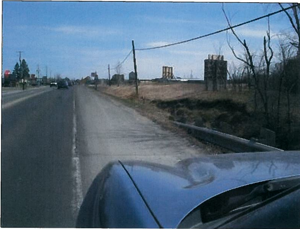
East Approach Rideau River (South Branch)
