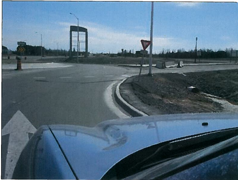
Colonnade Road Roundabout
