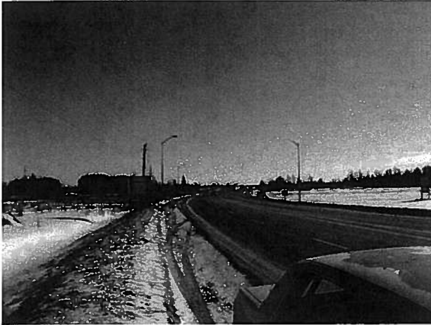
Plate 1: Looking south-east along CR43 at 416 interchange at undisturbed fallow fields beyond disturbed right-of-way
