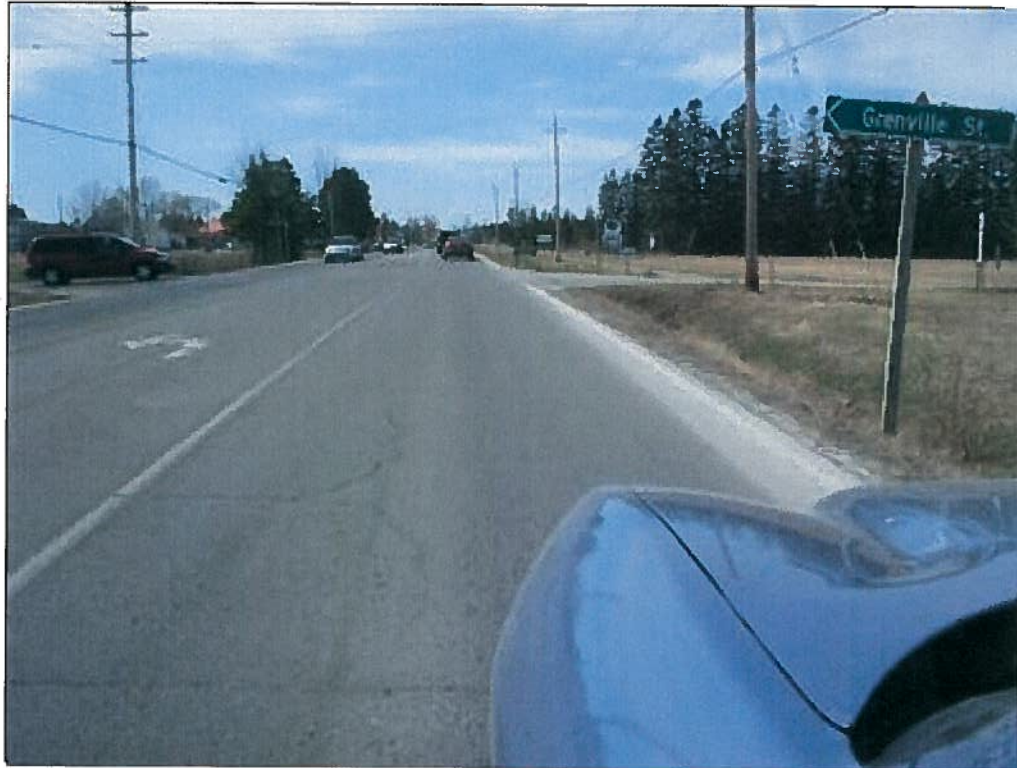
East of Grenville Street
