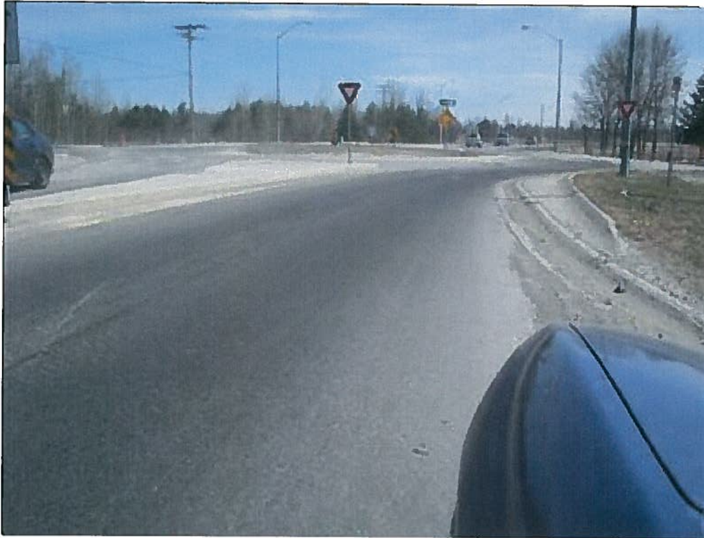
Wellington Street Roundabout
