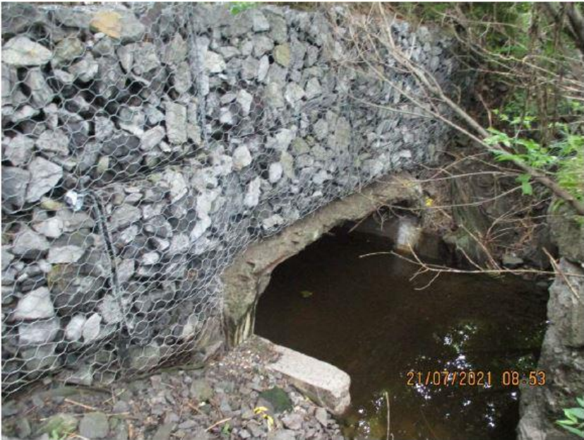
Figure 4-8: Example of Fair Condition Culvert – Grippen Creek Culvert (BCI 62.7)
