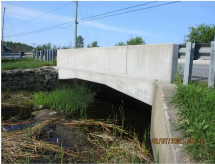
Figure 4-5: Example of Good Condition Bridge – MacIntosh Mills Bridge (BCI 91.1)
