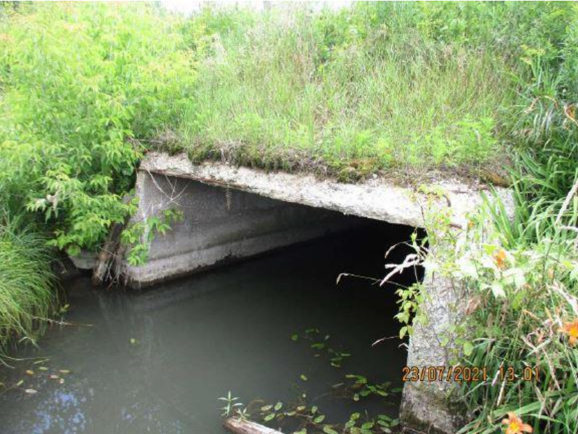
Figure 4-8: Example of Fair Condition Culvert – Grippen Creek Culvert (BCI 62.7)
