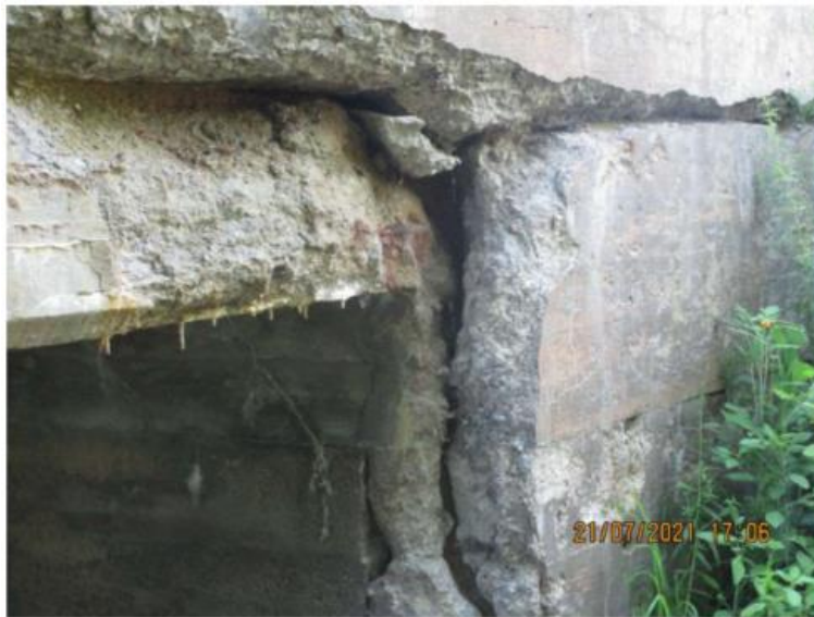
Figure 4-4: Example of Fair Condition Bridge – Smileys Bridge (BCI 64.9)
