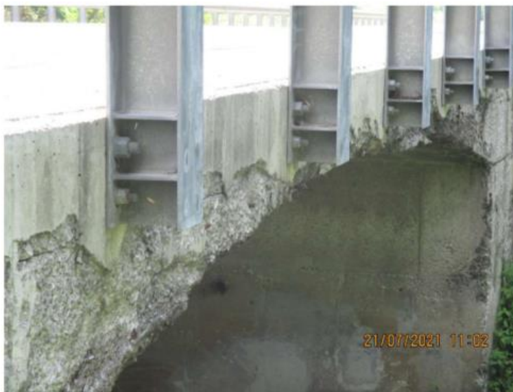
Figure 4-4: Example of Fair Condition Bridge – Smileys Bridge (BCI 64.9)
