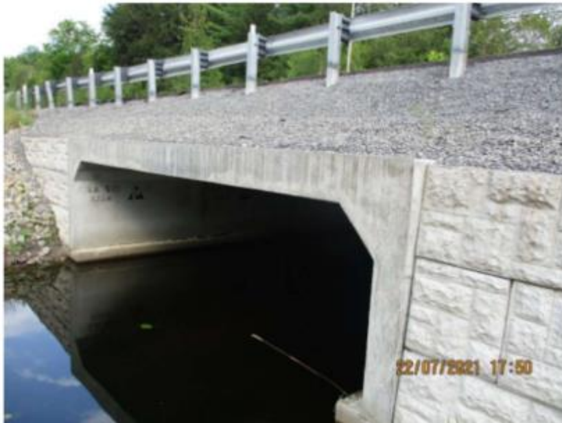
Figure 4-9: Example of Good Condition Culvert – Crosby Creek Culvert (BCI 93.4)
