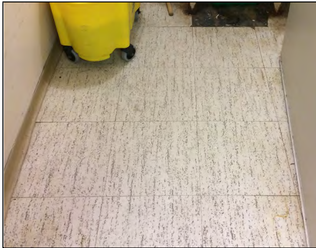
Photo 1: Asbestos-containing 12"x12" vinyl floor tiles beige with black dots (2.41% Chrysotile) and associated mastic (0.95% Chrysotile) observed in the custodian's closet. The mastic was exposed at the right corner.
