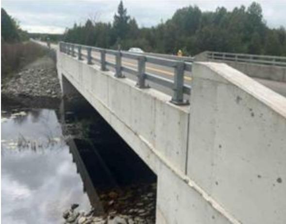
Very Good Bridge (Mud Creek)
