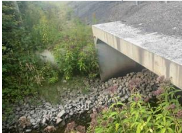
Good Culvert (Van Camp Drain)
