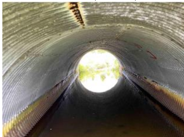
Fair Culvert (Fish Creek)
