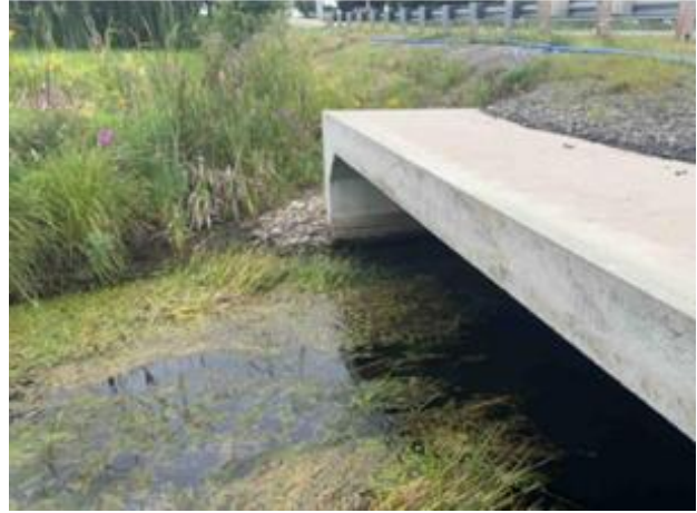
Very Good Culvert (Butler Creek)
