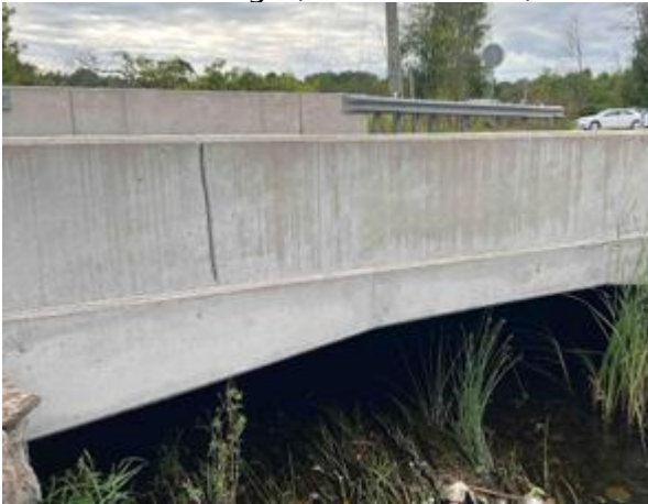
Good Bridge (MacIntosh Mills)
