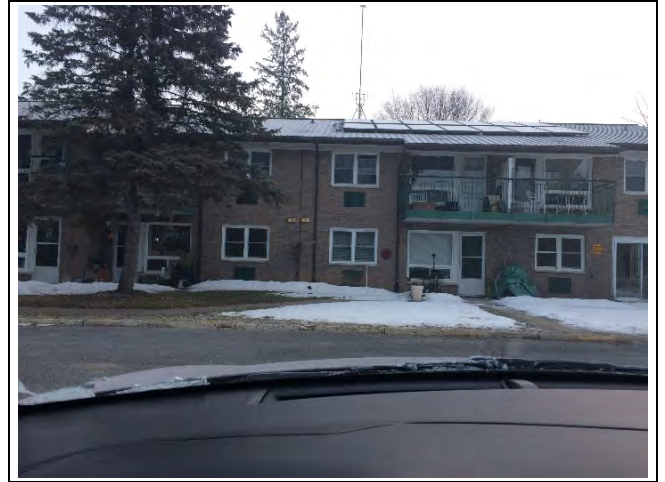
Photo 6: Presumed asbestos-containing roof caulking suspected to be present on the metal roof observed
