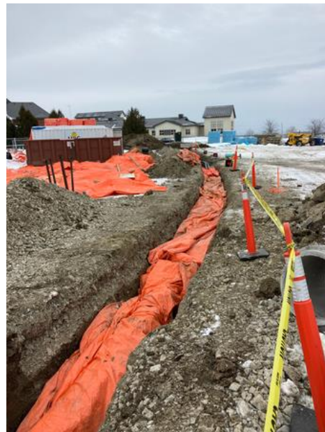
Excavation of building commenced and protected with insulated tarps
