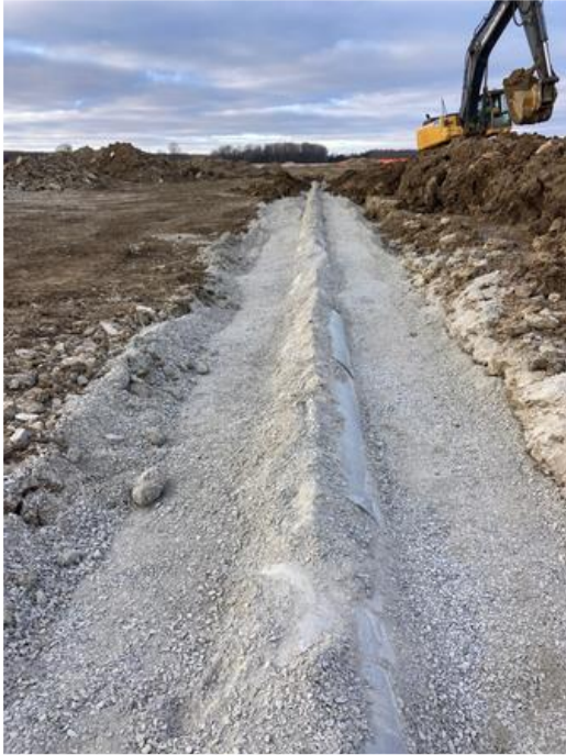
Backfill over piping
