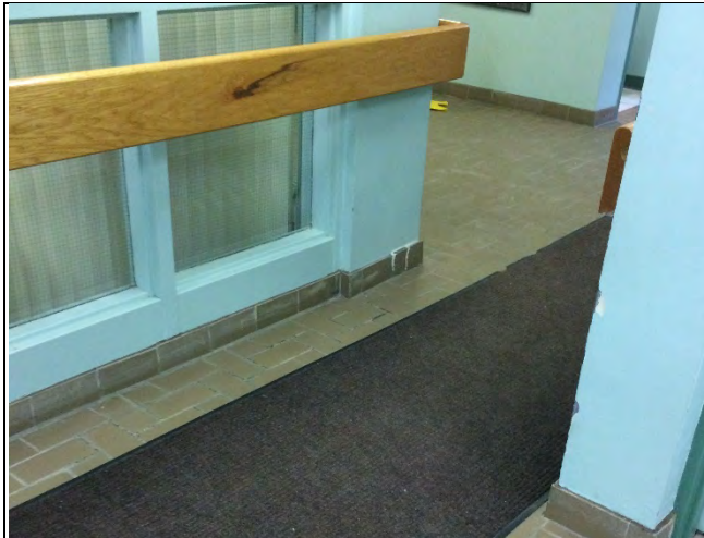
Photo 3: Asbestos-containing drywall joint-fill compound on the walls and presumed asbestos-containing ceramic tile grout and mortar/adhesive on baseboards and floor observed to be in good condition in the 1 st floor corridor.
