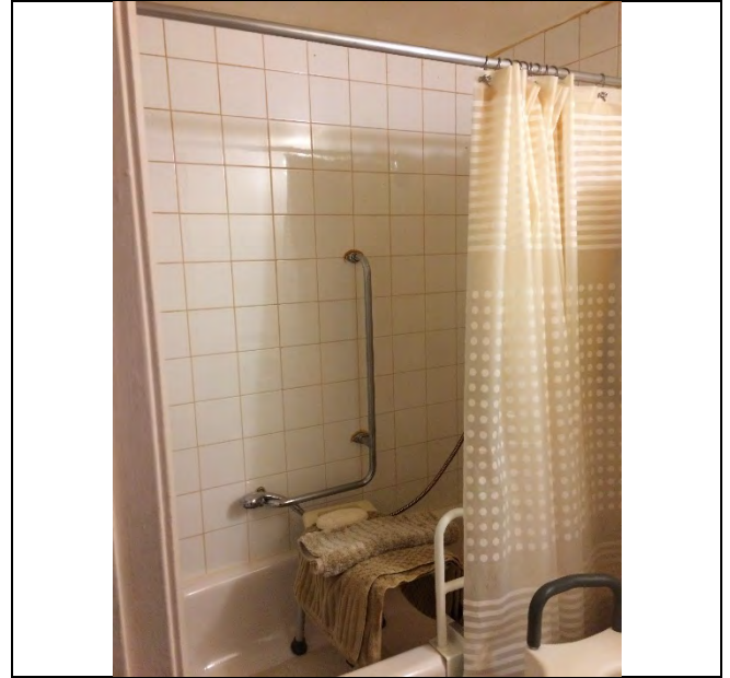
Photo 6: Presumed asbestos-containing ceramic tile grout and mortar/adhesive observed to be in good condition on walls in the washroom at unit 103.
