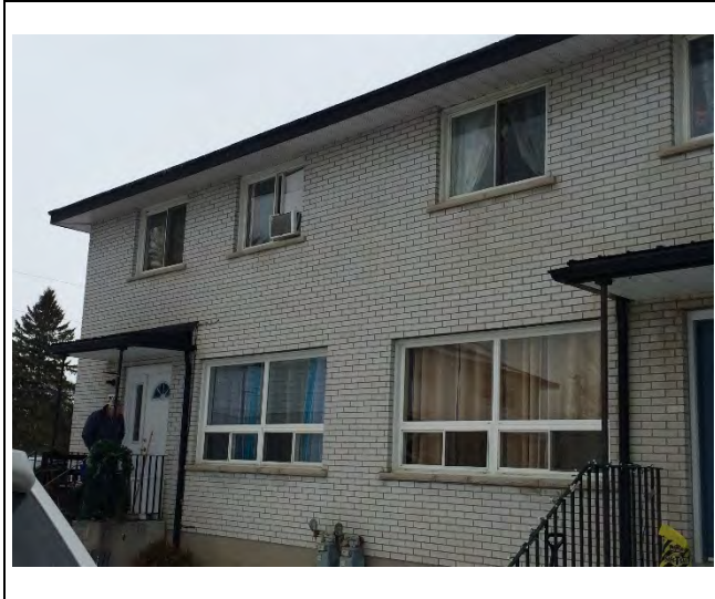
Photo 1: Presumed asbestos-containing brick mortar, roofing materials and roof caulking was observed to be present on the exterior of the house.
