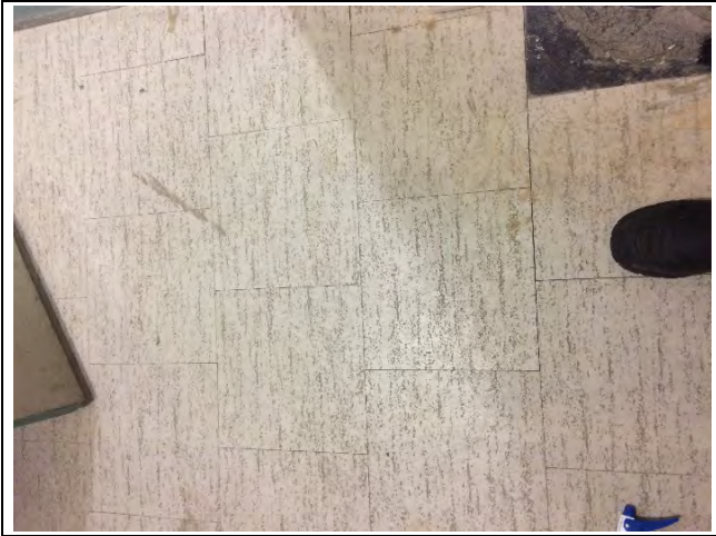
Photo 1: Asbestos-containing 12" x 12" vinyl floor tiles – beige with black spots (3.89% Chrysotile) in the communal storage room.
